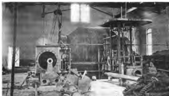
A. INSTALLING NEW HOIST AT LAKE MINE, 1911, U. S. GEOLOGICAL SURVEY.
